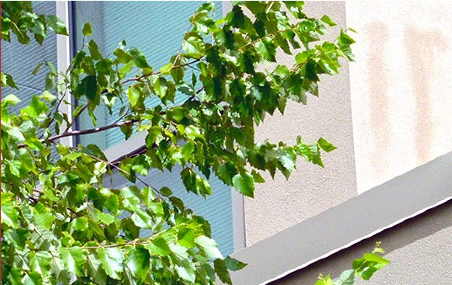
Photo Info : Water staining on face of wall at area with inconstant drainage plane
