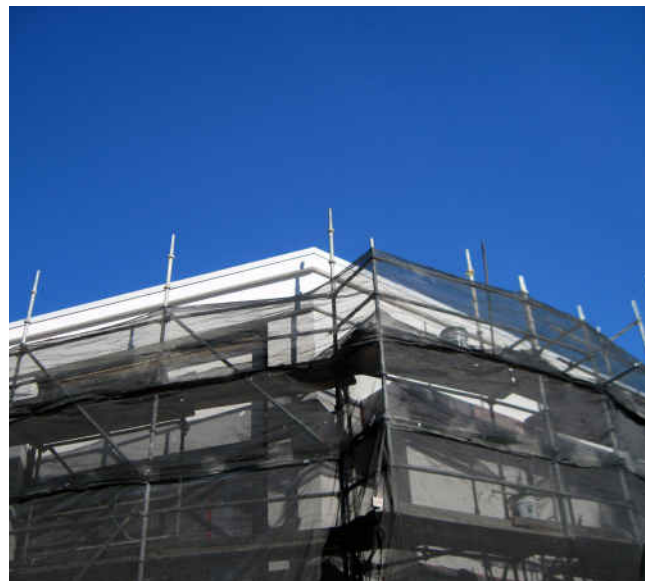
Photo Info : Tommy Bahamas Exterior Insulation and Finish System (EIFS) Underway.
