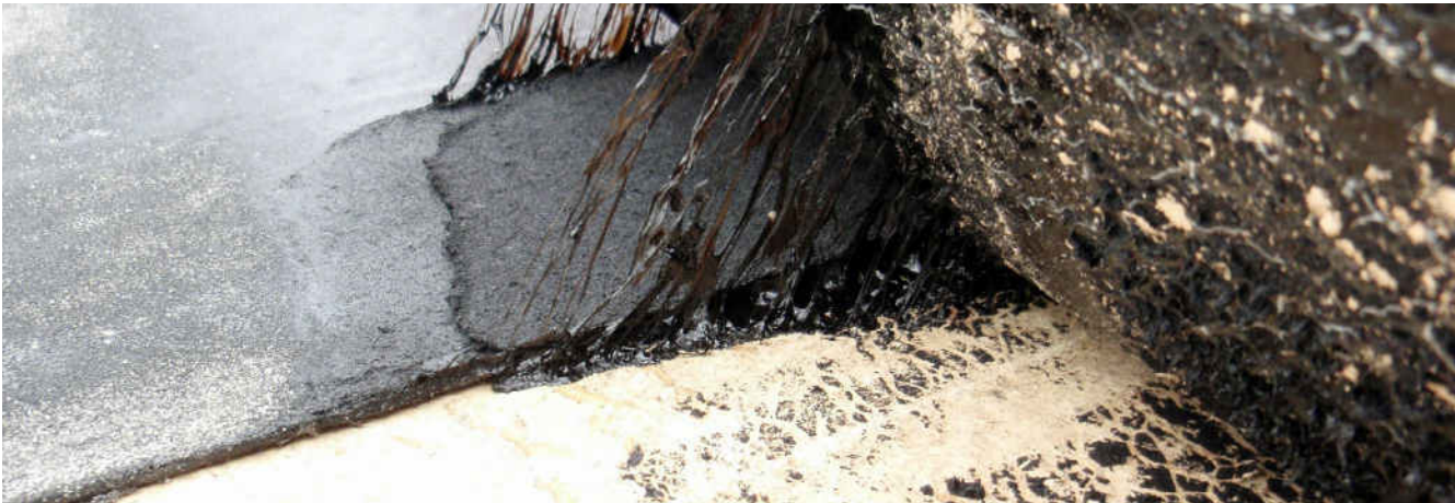
Figure 5: During proper heat application of torch applied membrane, the roll can be rolled back and “stringers” of modified asphalt can be observed. This is an indicator of adequate heat at the point of application.
