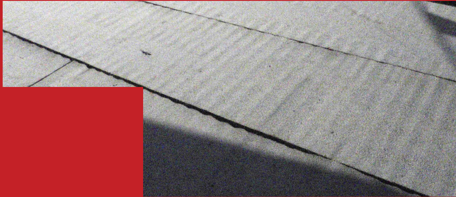
Figure 1: Washboarding observed on a Torch Applied Roof Membrane.
