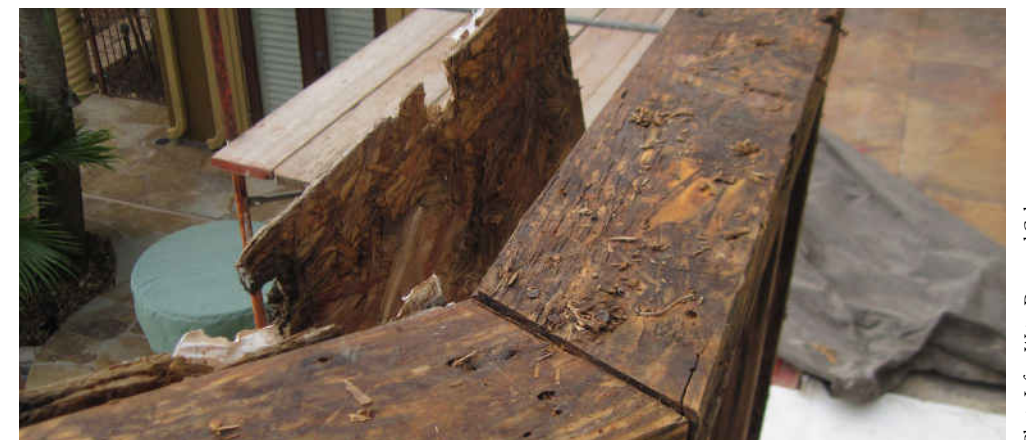
Photo Info : Water Damaged Column.
