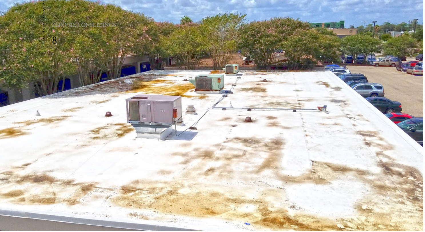
Photo Info : Lack of adequate slope (minimum \frac{1}{4} " per foot) causing ponding which destroys the membrane
